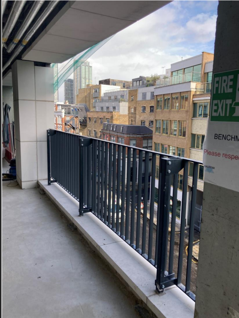
Balustrade & GRC installation
