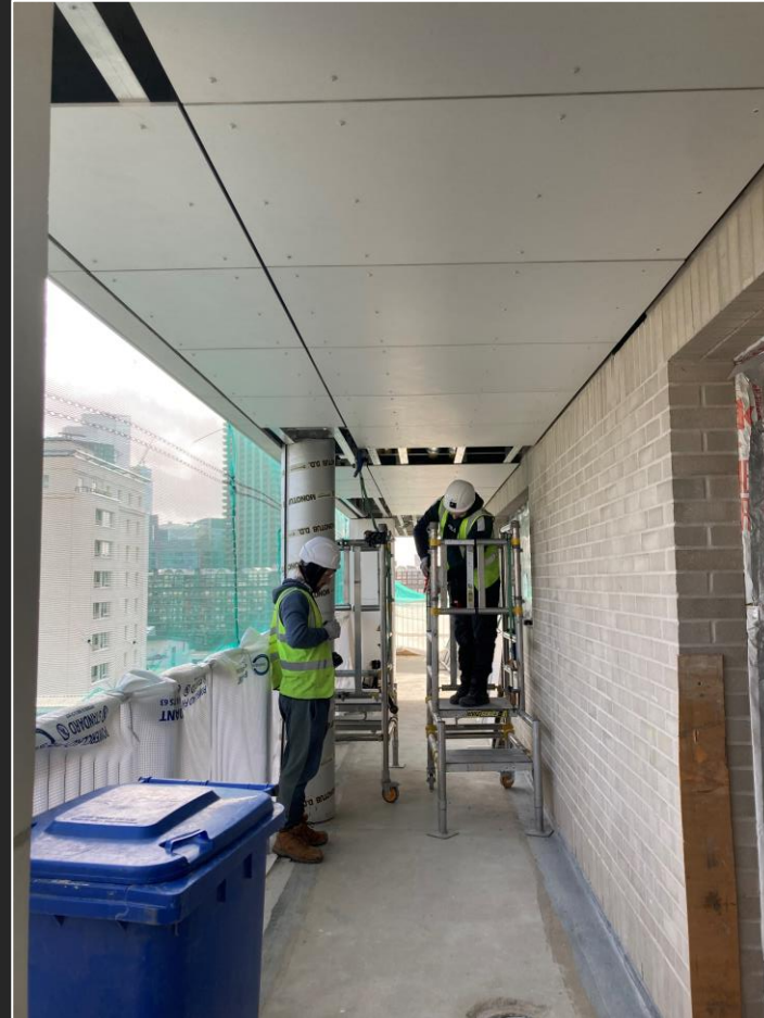
Walkway soffit installation
