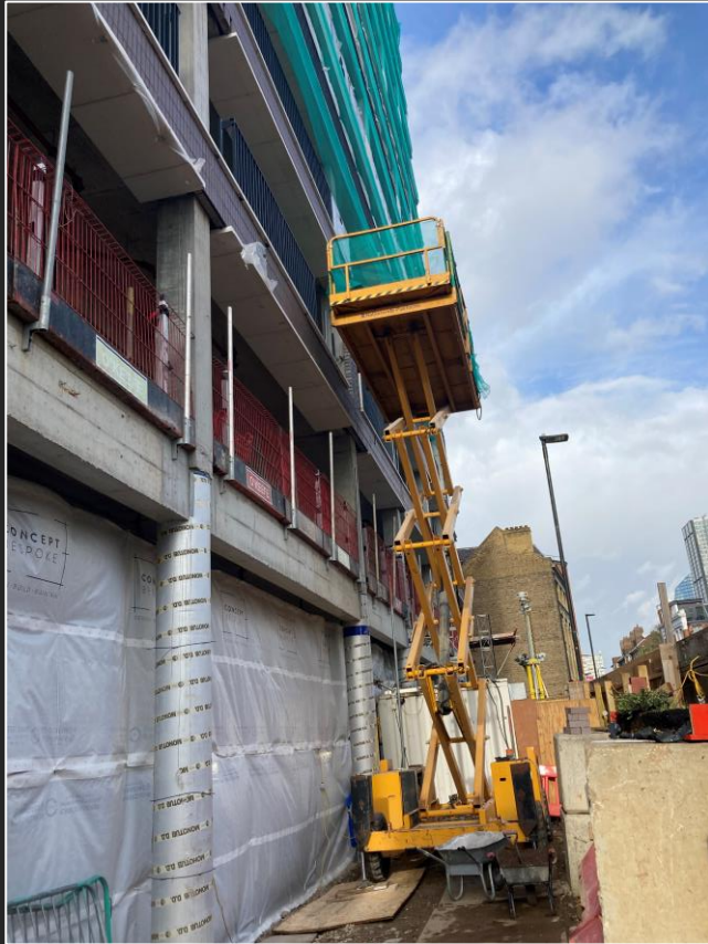
Scaffold removal and MEWP brickwork installation
