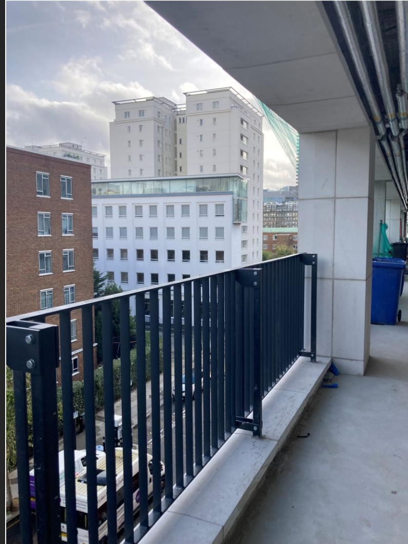
Balustrade & GRC installation
