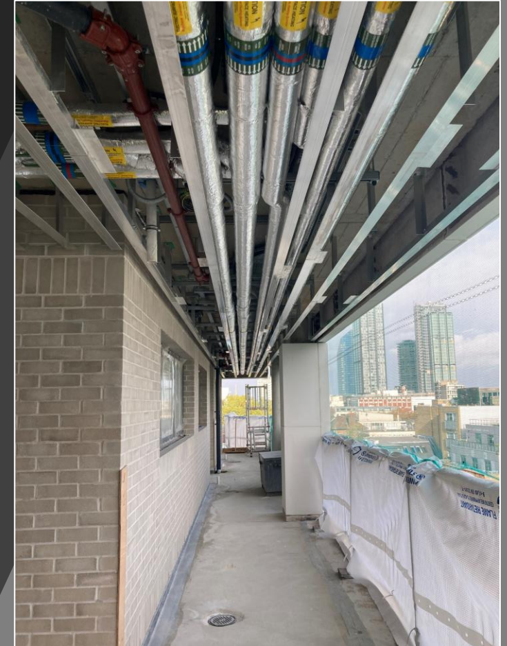
Balcony / walkway soffit bracketry ongoing
