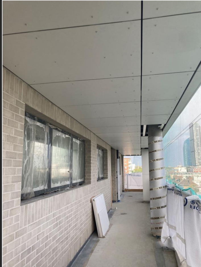
Walkway soffit installation
