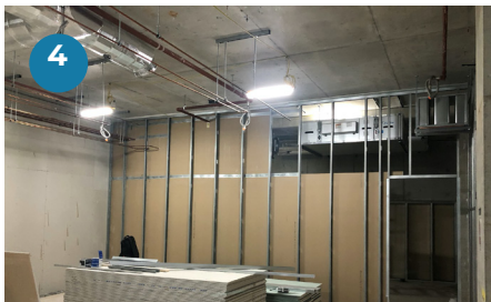
Ground floor first fix drylining (After the removal of old temporary welfare)
