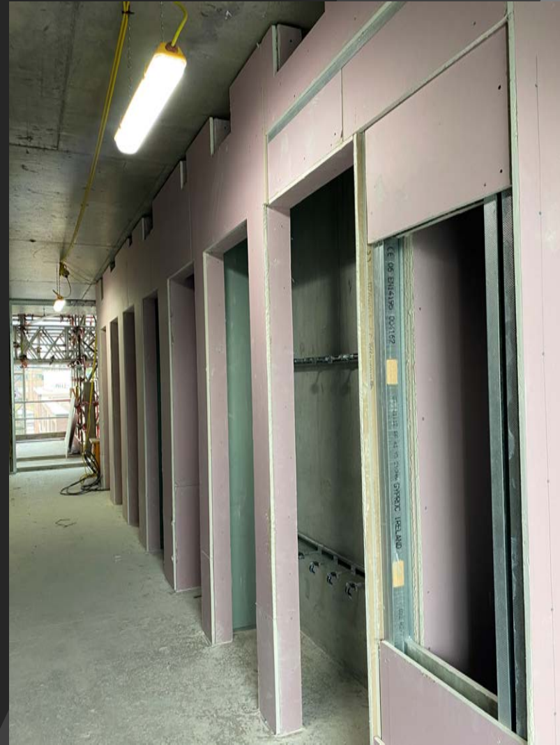
Riser walls installed
