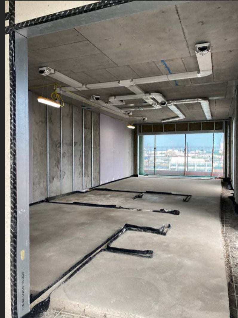
Screeding and ducting completed
