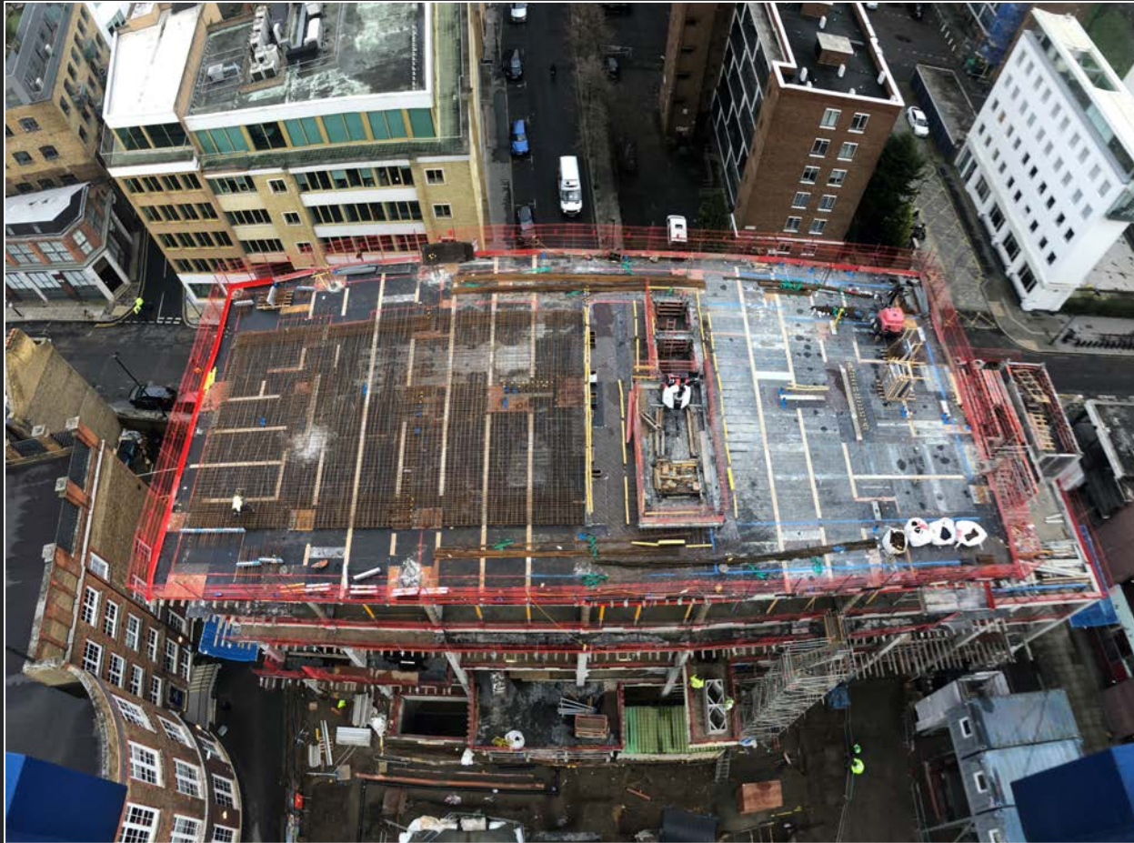
Residential progress – sixth floor slab preparation
