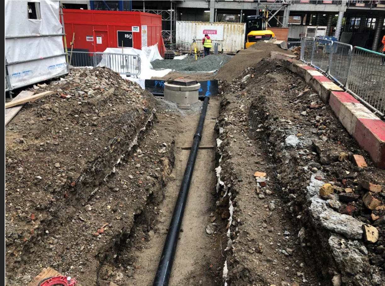
Sprinkler main progress
