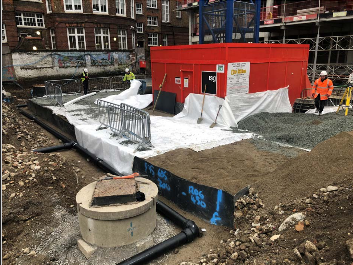
Attenuation tank installation progress
