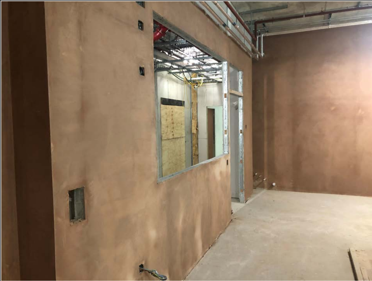
Main school building drywall and plastering
