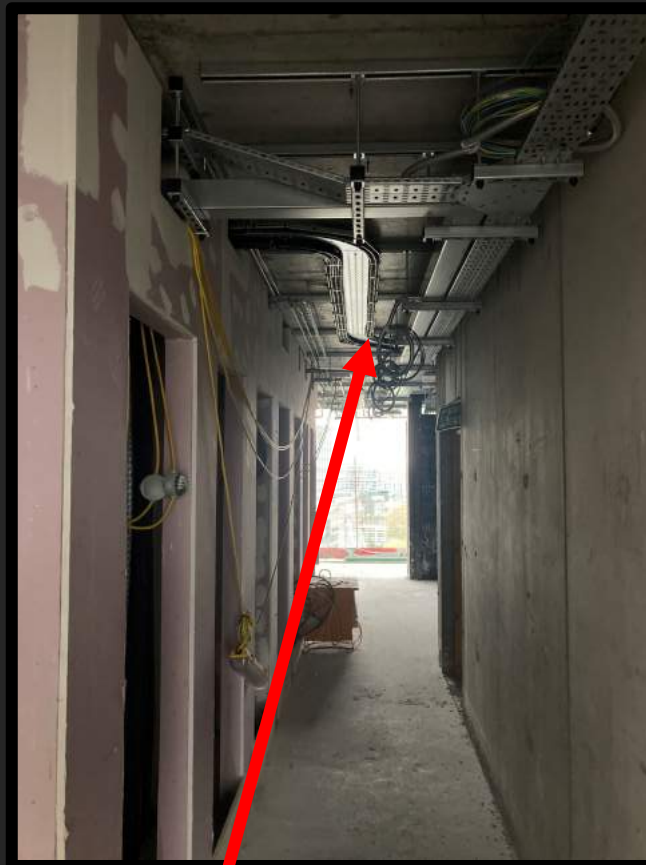
High level 1 st fix M&E installation ongoing throughout.
