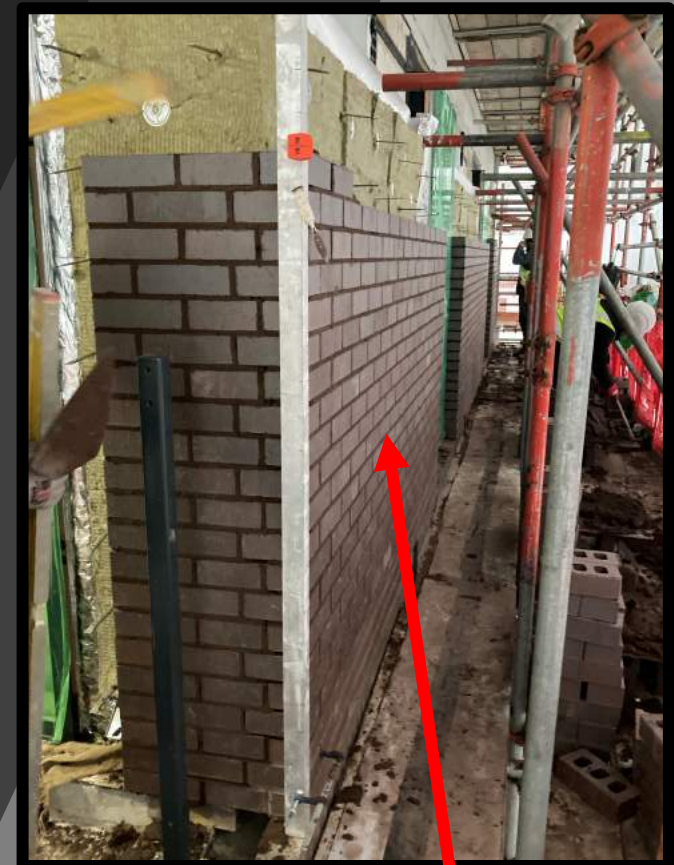
External brickwork façade installation.
